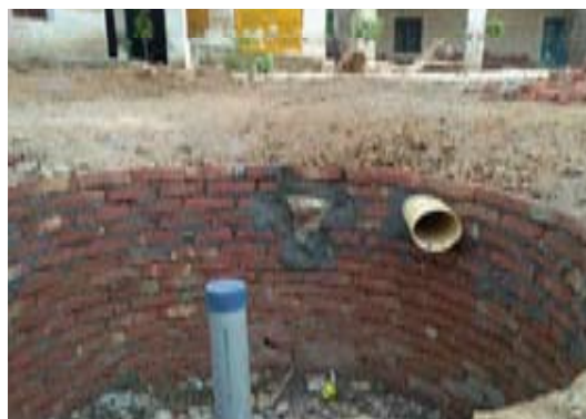
Rain water harvesting structure at Gajraula
