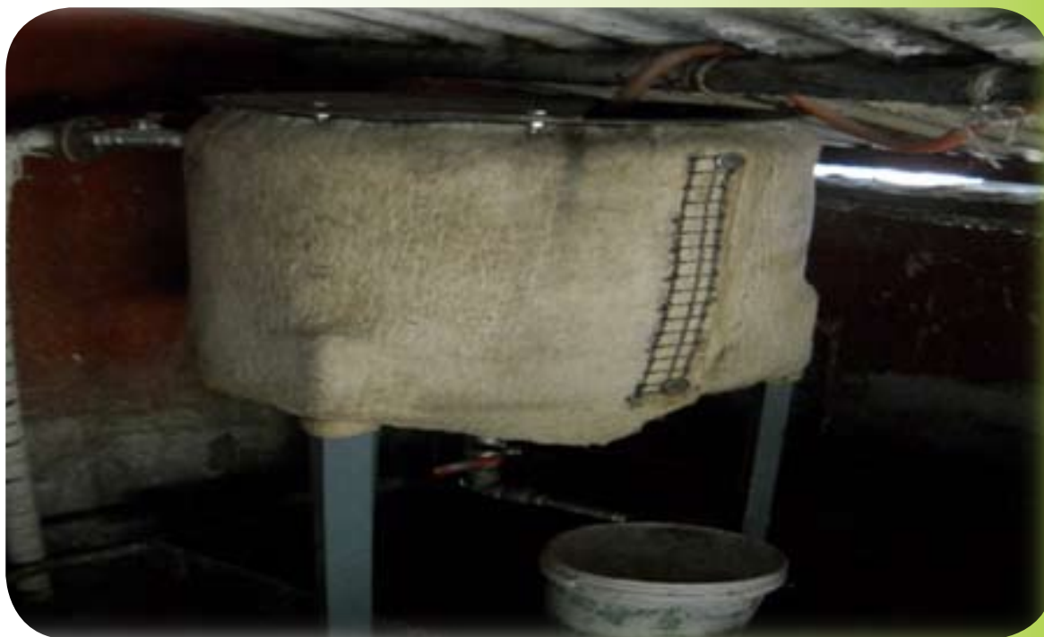
At Sahibabad, small vessel is designed and installed for heating the water. Hot water is used for cleaning of filter in place of direct steam which is safe and easy to operate.
