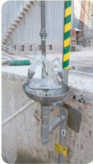
New eye wash showers installed in plant acid storage area and QC laboratory
