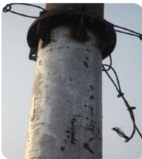
At Sahibabad plant, strengthening of Boiler stack carried out.
