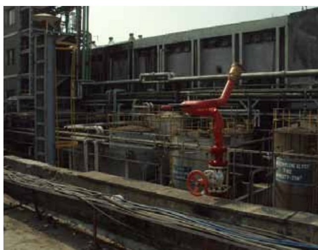
At Gajraula, Fire hydrant monitor provided for flammable chemicals (IPA & VAM) storage tanks.
